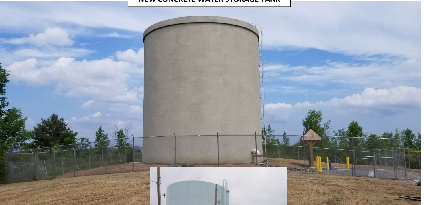
NEW CONCRETE WATER STORAGE TANK
