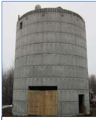
TANK PEDESTAL ALMOST COMPLETE
