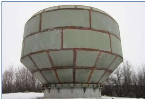
TANK STORAGE PARTIALLY COMPLETED
