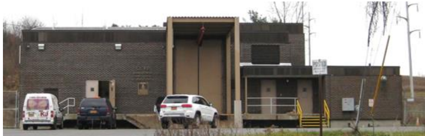
Eastern Pumping Station and Chlorination Building
