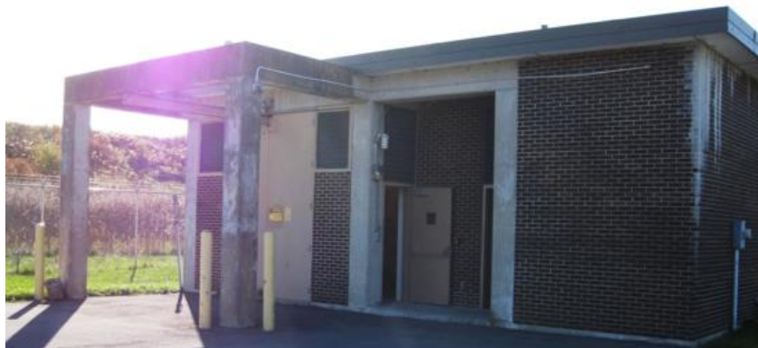
Western Chlorination Building
