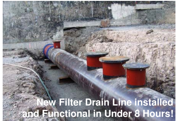
Excavation Work for New Filters
